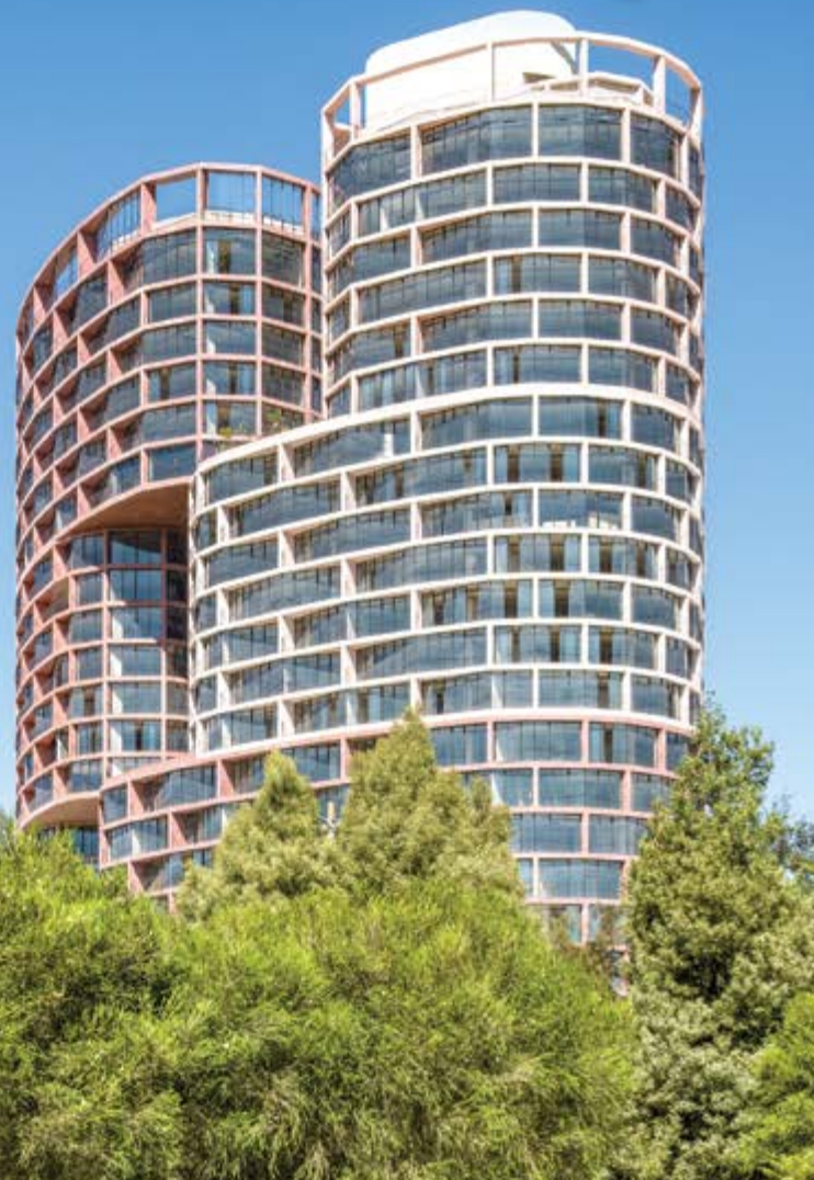
» EPIQ, 24 pisos. Quito, Ecuador. by @uribeschwarzkopf + BIG @big_builds, Bjarke Ingels @bjarkeingels Photography by: Bicubik Photo @Bicubik.photo
